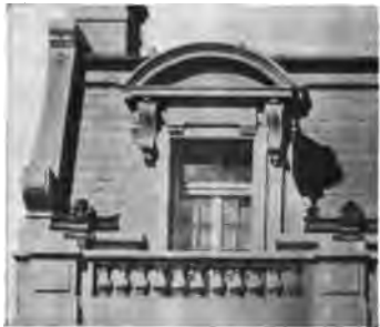
DORMER WINDOW WITH CURVED PEDIMENT, IN A MANSARD ROOF.
